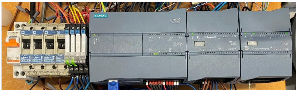
Figura 2 - PLC SIMATIC S7-1200 CPU 1215C AC/DC/RLY
